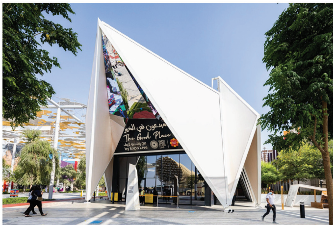
Expo Live Pavilion - Expo2020 Dubai Emergency Lighs: 50 | Exit Lights: 10 | Control Panel: 6
