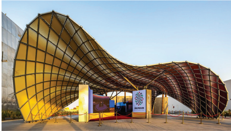
Iraq Pavilion - Expo2020 Dubai Emergency Lighths: 25 | Exit Lights: 10 | Control Panel: 3
