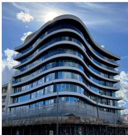
University Tower - Debrecen, Hungary Emergency Lighths: 46 | Exit Lights: 104 | Control Panel: 1
