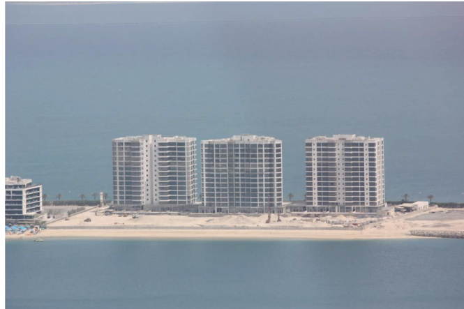
3 Commercial and Residential buildings - Palm Jumeirah, Dubai Emergency Lighths: 1000 | Exit Lights: 250 | Control Panel: 6
