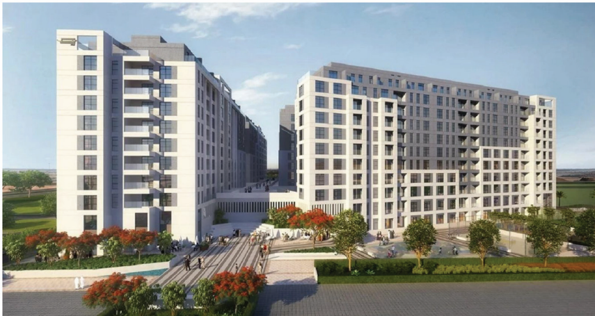
Commercial Buildings - Al Mamsha, Sharjah Emergency Lighths: 1400 | Exit Lights: 600 | Control Panel: 91
