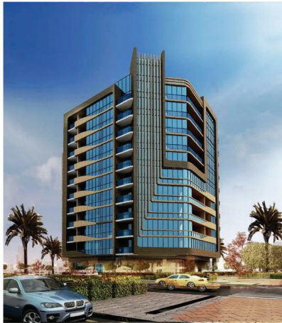
Residential Building - Nadd Al Hamer, Dubai Emergency Lighths: 300 | Exit Lights: 125 | Control Panel: 6
