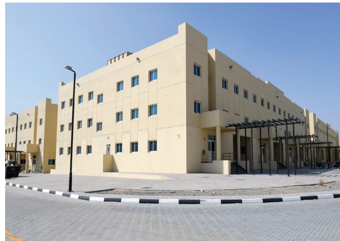
Labor Accomodation - Dubai Emergency Lighths: 250 | Exit Lights: 100 | Control Panel: 9
