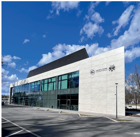
University of Debrecen E-Learning Center - Hungary Emergency Lighths: 123 | Exit Lights: 118 | Control Panel: 1
