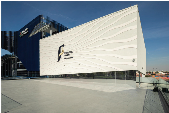
Firdaus Pavilion - Expo2020 Dubai Emergency Lighs: 125 | Exit Lights: 50 | Control Panel: 3
