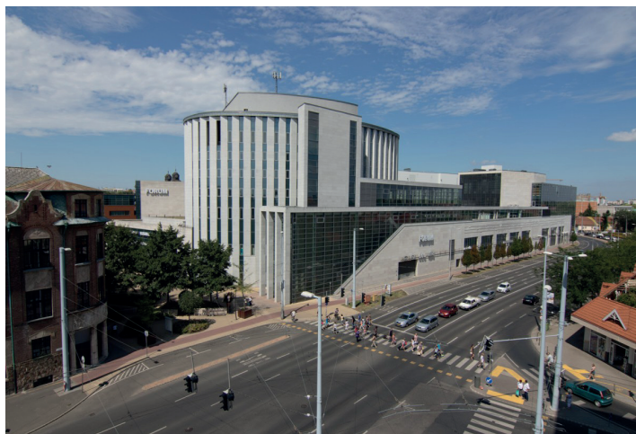
Csokonai Fórum - Debrecen, Hungary Emergency Lighths: 314 | Exit Lights: 237 | Dynamic Lights: 36 | Control Panel: 5
