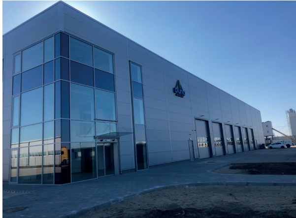
DunaGroup Building - Hungary Emergency Lighths: 32 | Exit Lights: 60 | Control Panel: 1
