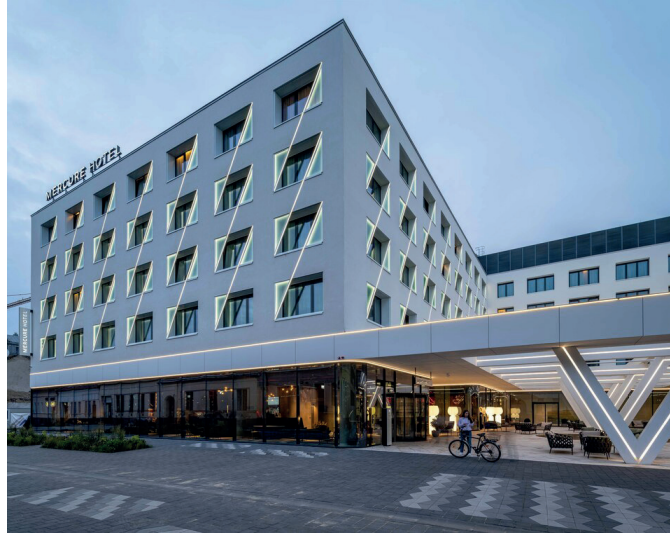
Mercure Hotel - Debrecen, Hungary Emergency Lighths: 222 | Exit Lights: 251 | Control Panel: 5
