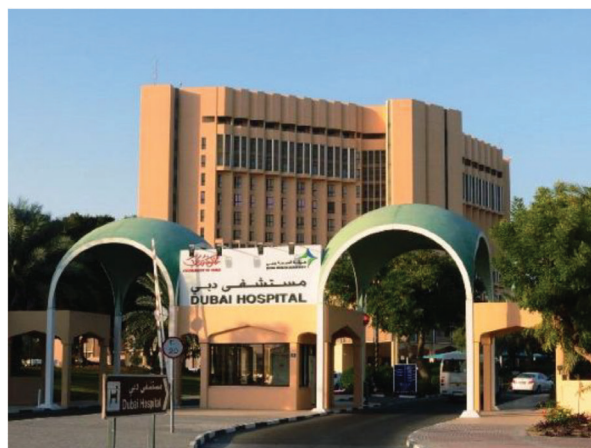
Outpatient Extension Building - Dubai Hospital Emergency Lighths: 1500 | Exit Lights: 500 | Control Panel: 100
