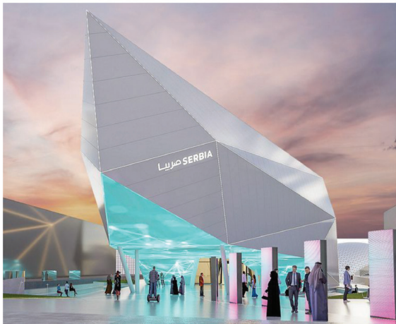
Serbia Pavilion - Expo2020 Dubai Emergency Lighths: 75 | Exit Lights: 25 | Control Panel: 1
