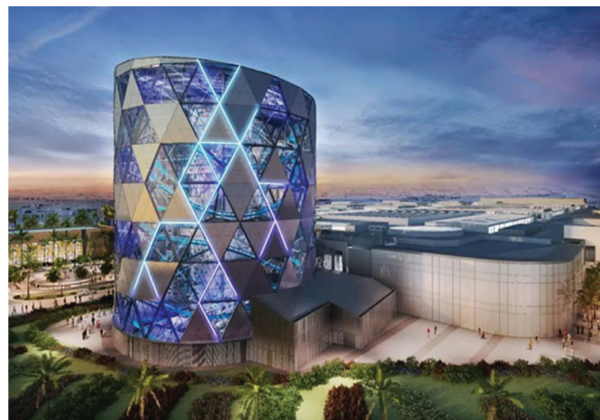
Dubai Hills Mall Indoor Coaster Emergency Lighths: 400 | Exit Lights: 150 | Control Panel: 4
